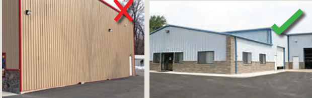
Left, a metal-faced (or concrete panel) building devoid of any architectural merit or character. Right, an industrial building using stone as a base material and metal siding making up to 75% of the remaining facade.
