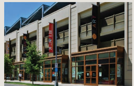
Design for a parking structure along a public street should provide visual interest compatible with adjacent developments and is encouraged to provide occupable spaces along the street level.
