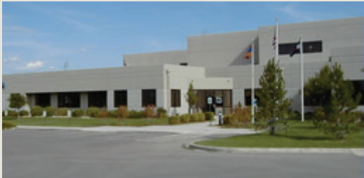
Variations in facade depth and heights for industrial buildings to break up long monotonous walls
