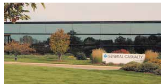
Commercial (QBE Office Campus)
