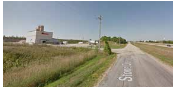
Stone Quarry Rd along USH 151
