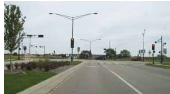
Principal Arterial Grand Ave. at Hoepker Rd.
