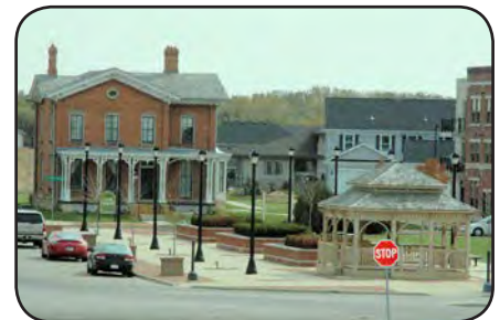
Adam and Mary Smith House Pre and Post Relocation
